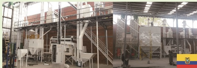
5T/H Rice Seed Processing Plant in Ecuador
