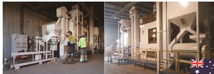
10T/H Wheat and Barley Seed Processing Plant in Australia
