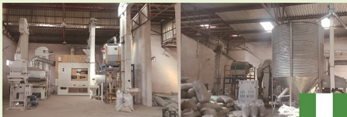
10T/H Sorghum Cleaning Plant in Nigeria
