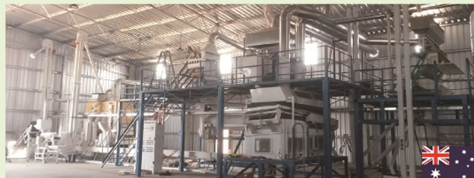
1.5T/H Quinoa Seed Processing Plant in Australia
