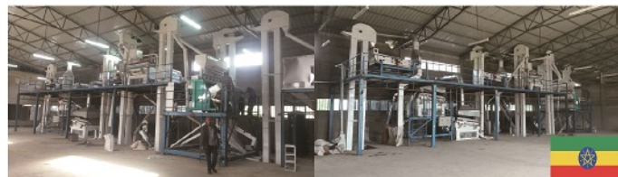
8T/H Pulses and Sesame Cleaning Plant in Ethiopia
